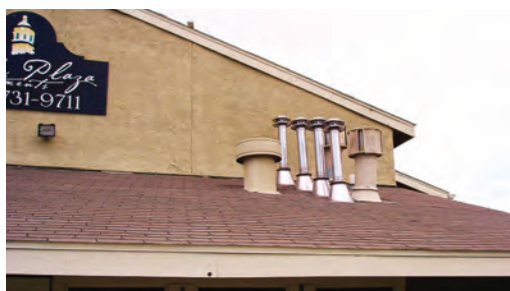
Four vertical 5" vent terminations through the roof top.
